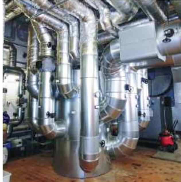
Zortström Multi-H 4-stufig Durchmesser 1.300 mm
