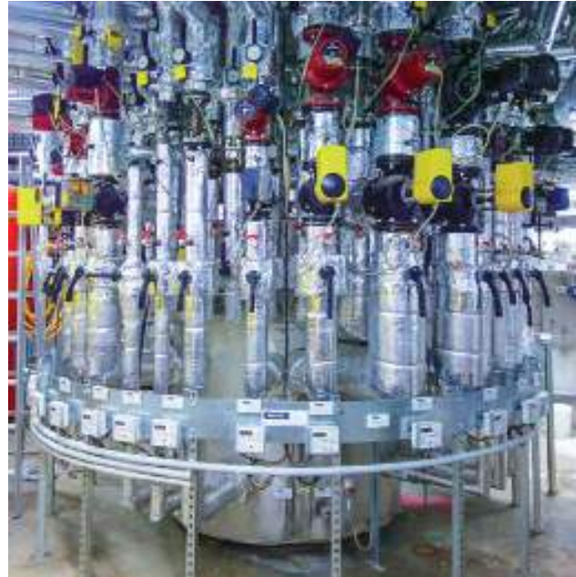
Zortström Multi-H 4-stufig Durchmesser 1.500 mm
