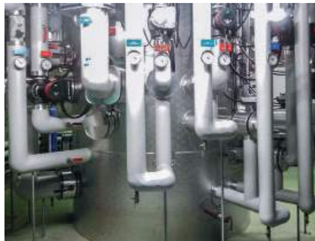
Zortström Multi-H 5-stufig Durchmesser 1.900 mm
