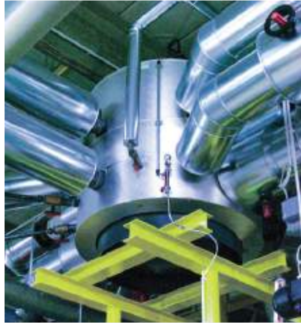
Zortström Multi-H 2-stufig Durchmesser 900 mm
