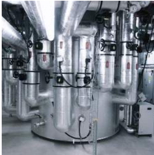
Zortström Multi-H 6-stufig Durchmesser 2.000.mm
