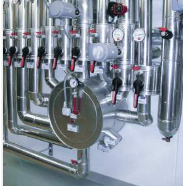
Zortström Multi-H 2-stufig Durchmesser 900 mm
