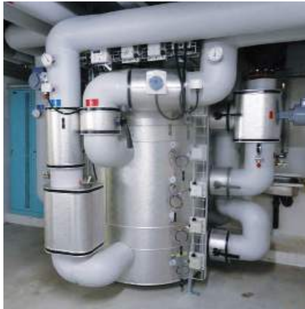
Zortström Multi-H 5-stufig Durchmesser 1.000 mm
