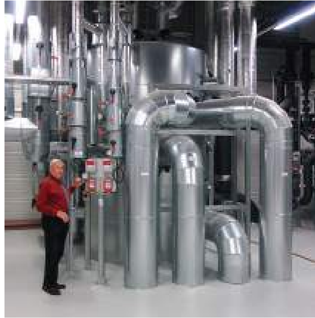
Zortström Multi-H 5-stufig Durchmesser 2.200 mm
