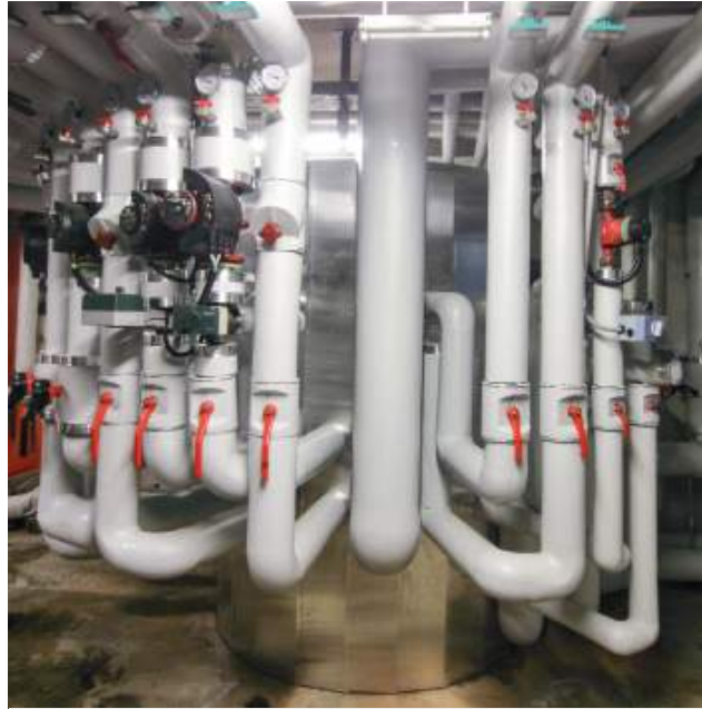
Zortström Multi-H 5-stufig Durchmesser 1.200 mm
